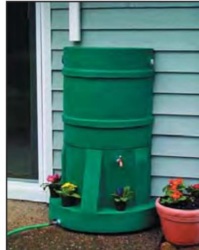
The purpose of these BMPs is not to capture 100 percent of the runoff from all storm events, but to capture the runoff from the first one-half to one inch of rainfall, which represents the most frequent storms within the San Diego region. A typical volume of rainfall targeted for capture (retention or re-use) from a 2,000 square foot home with a two car garage and 20 foot long driveway is as follows:
